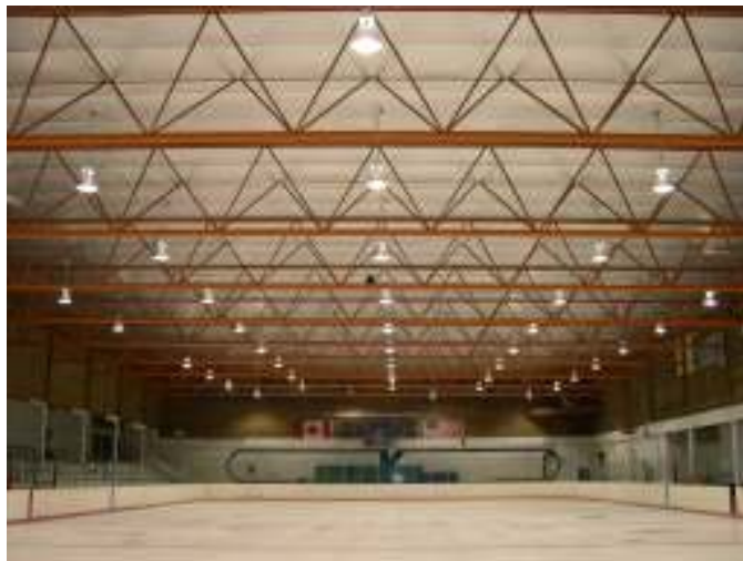
The benefits to the residents of Burnaby went beyond energy savings. Local hockey players and ice skaters were impressed with the improved lighting levels and harder ice surface in the retrofitted Kensington Arena.
